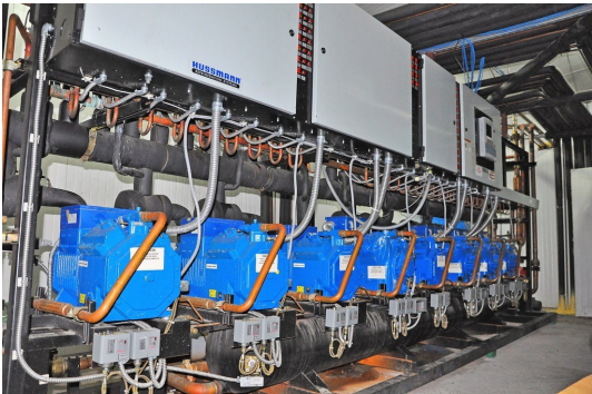
A Typical Row of 8 Compressor Units Found in Every Supermarkets
